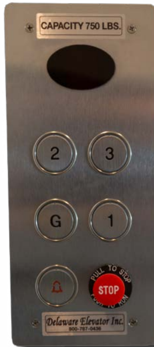
Control Operating Panel
